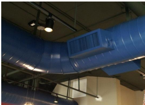
The exposed spiral ductwork on the first floor
