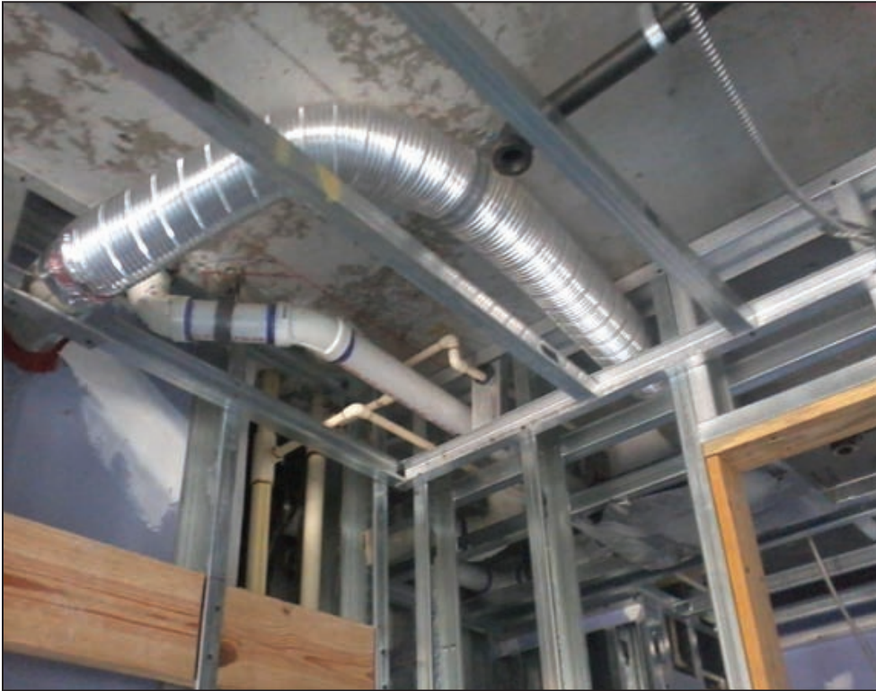
all trades coordinated above the bathroom ceiling
