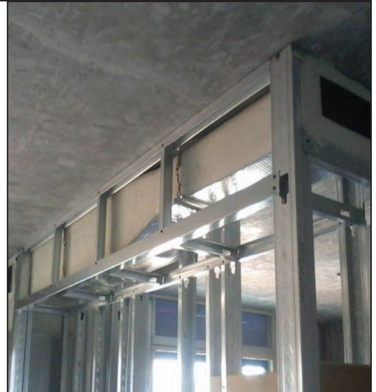
fiberglass room duct system, 1120 required
