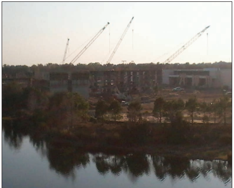
next building rising
