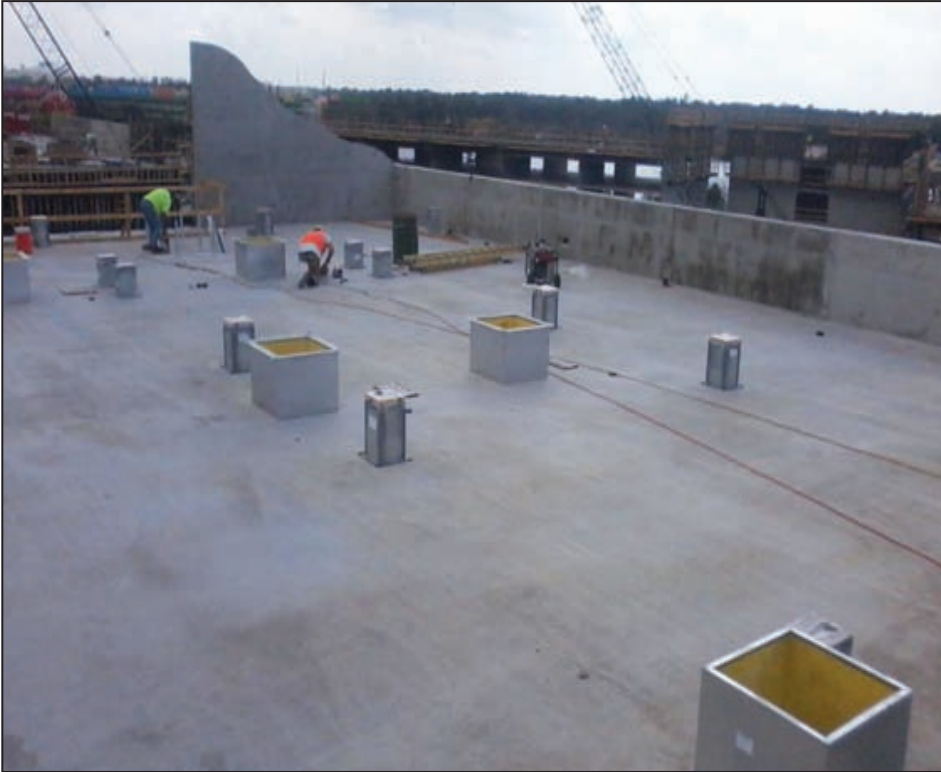
roof curb lay-outs and the next building rising in the background
