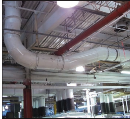
Relocated duct to facilitate installation of new AHU equipment and supports
