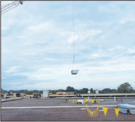
Equipment removal prior to new installation
