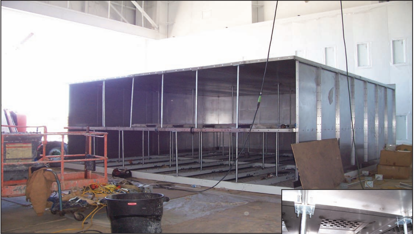
supply plenum being assembled on the ground
