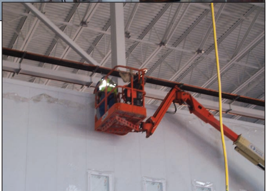
standing up walls of paint booth
