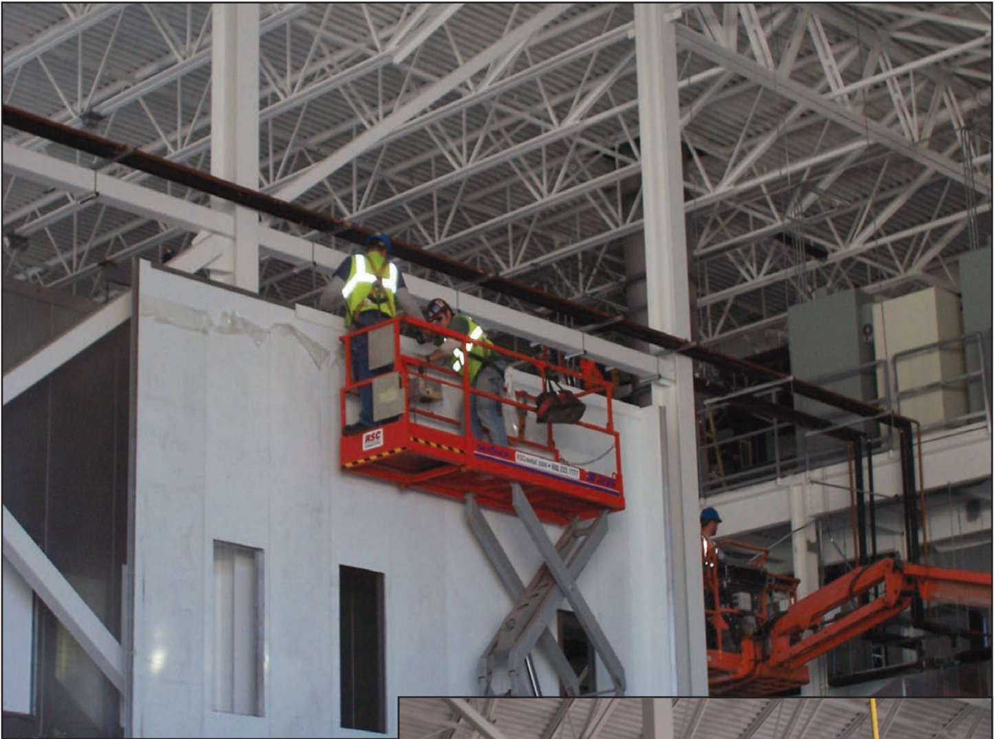
walls and panels for paint booth
