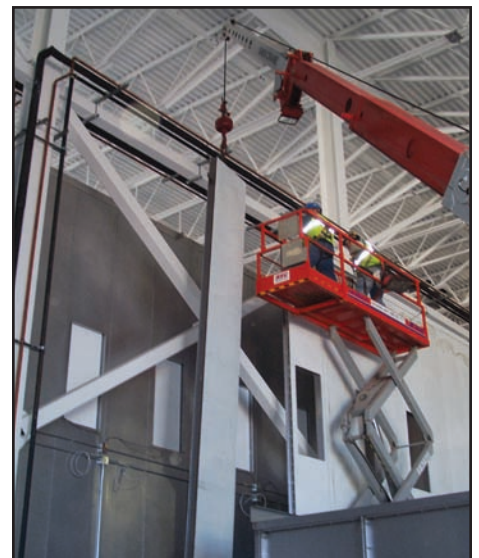
walls of paint booth
