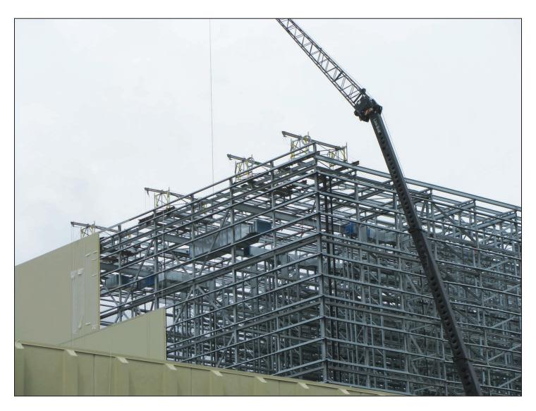
With close coordination and working together with J. Raymond, the General Contractor, and Schaefer Systems International, Inc., the steel erectors, Lapin flew its ductwork up with the steel.
