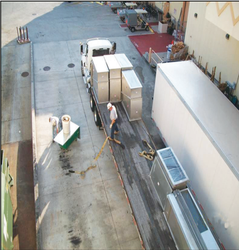
unloading trailer preparing for crane lifts
