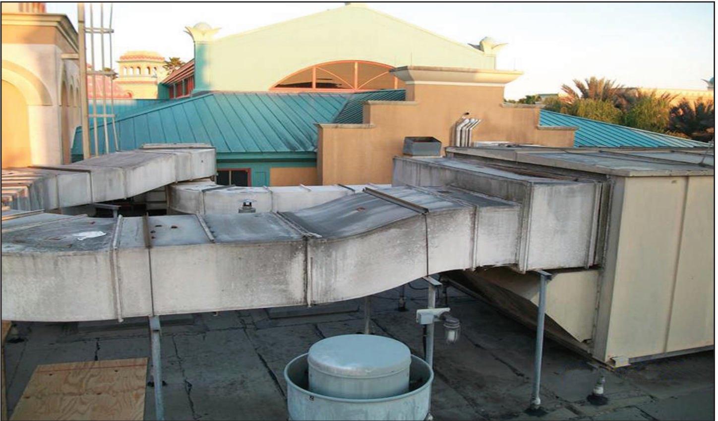
old single wall lined duct before demolition
