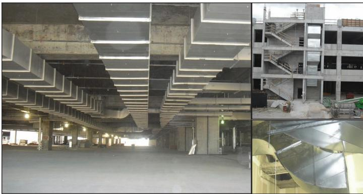
One challenge to the coordination of the project was the fact that no floor, where cars are driven, is level. In most areas, the floor slopes 14 inches over 60 feet and the floor above does not always pitch in the same direction. This made coordinating the ductwork to fit inside the allotted space tedious, as there is a 10 foot above finish floor clearance requirement for emergency vehicles. Many of the beams were 5.5 feet deep, with most of the duct 80 x 36 inches.
