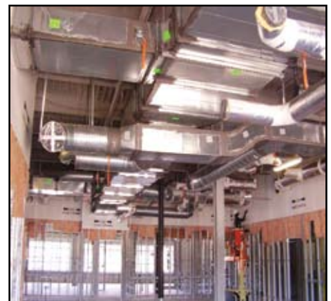
above ceiling rough-in complete
