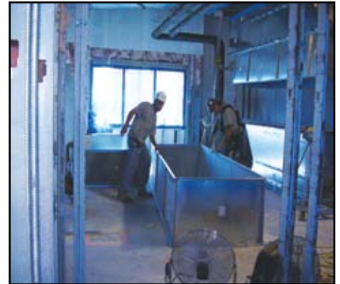
riser duct tie-in
