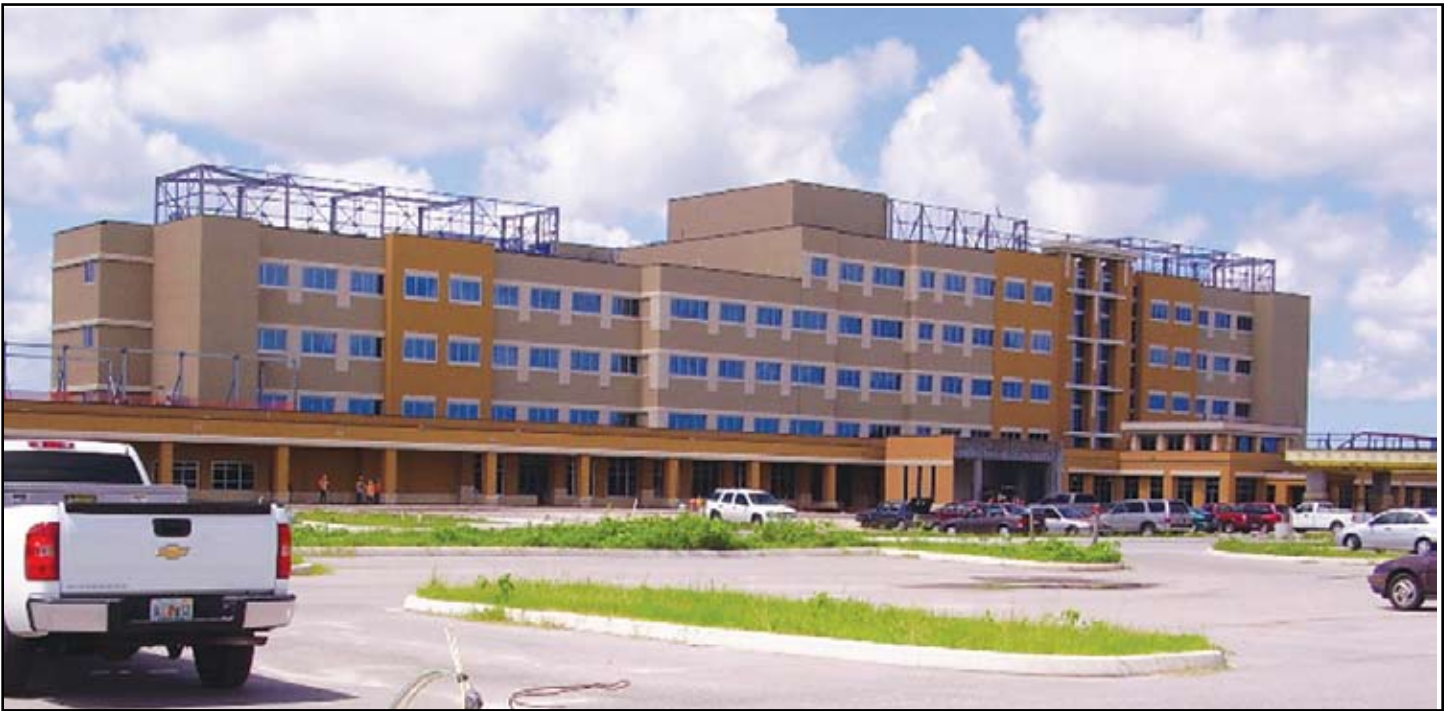
front view of building
