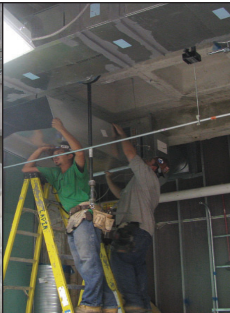
Installing ductwork in existing hospital
