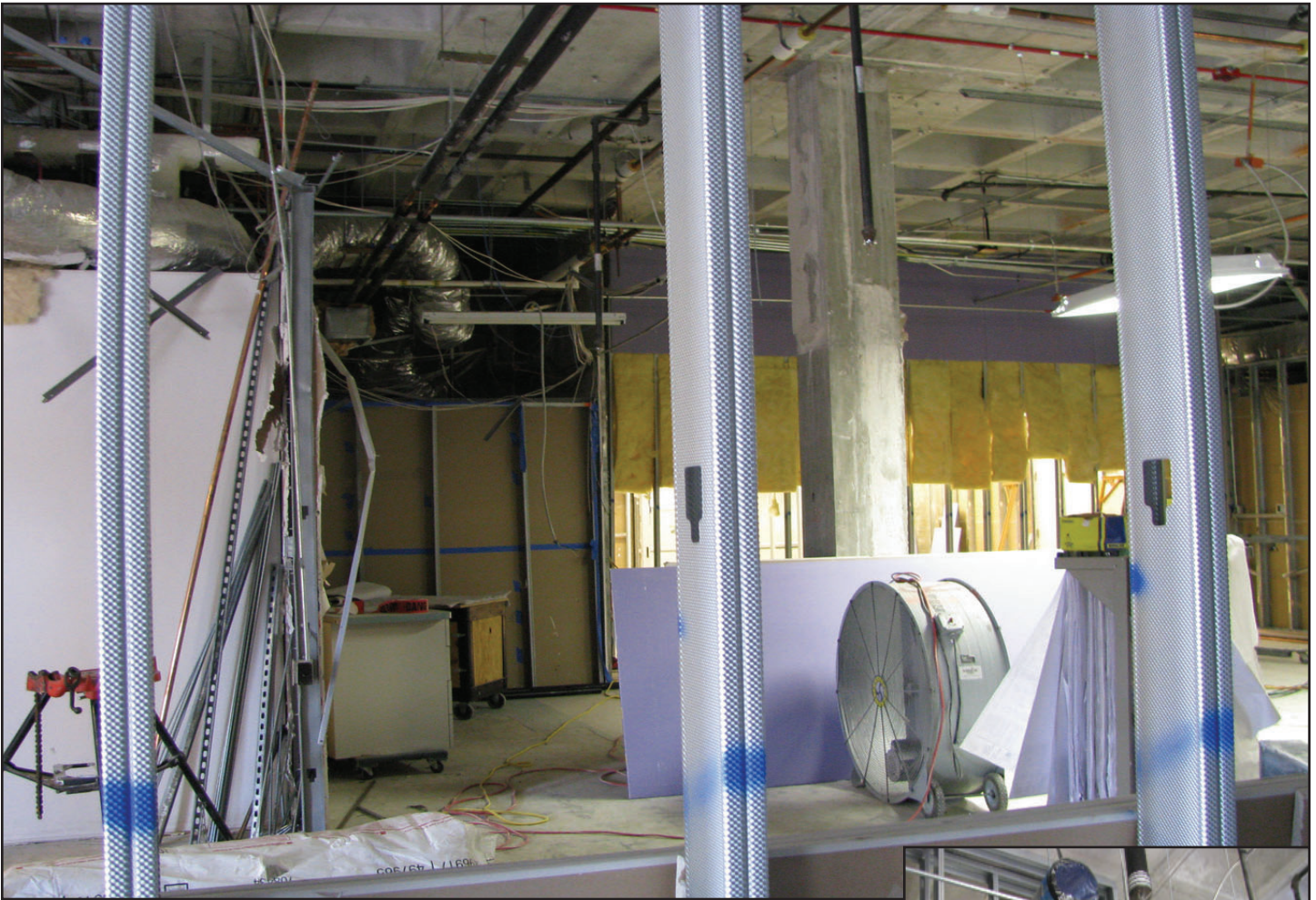
Demolition going on
