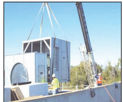
SETTING RETURN AIR EXHAUST UNITS SECTIONS
