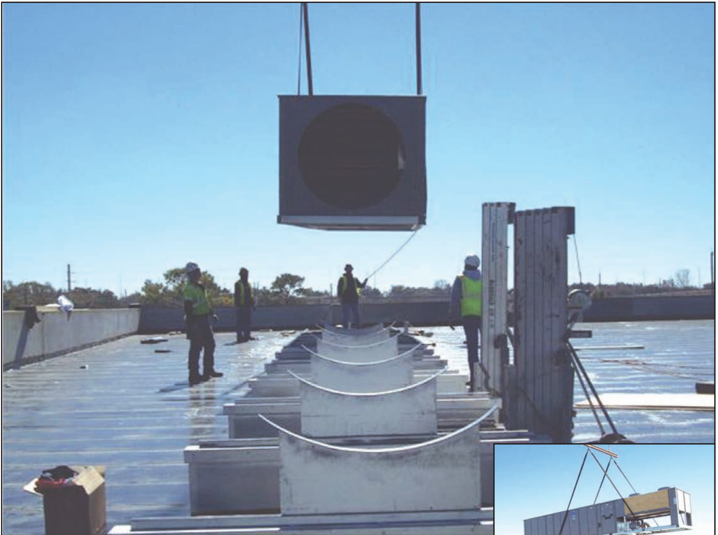
HOISTING 11,000 LB MAKE UP AIR UNIT
