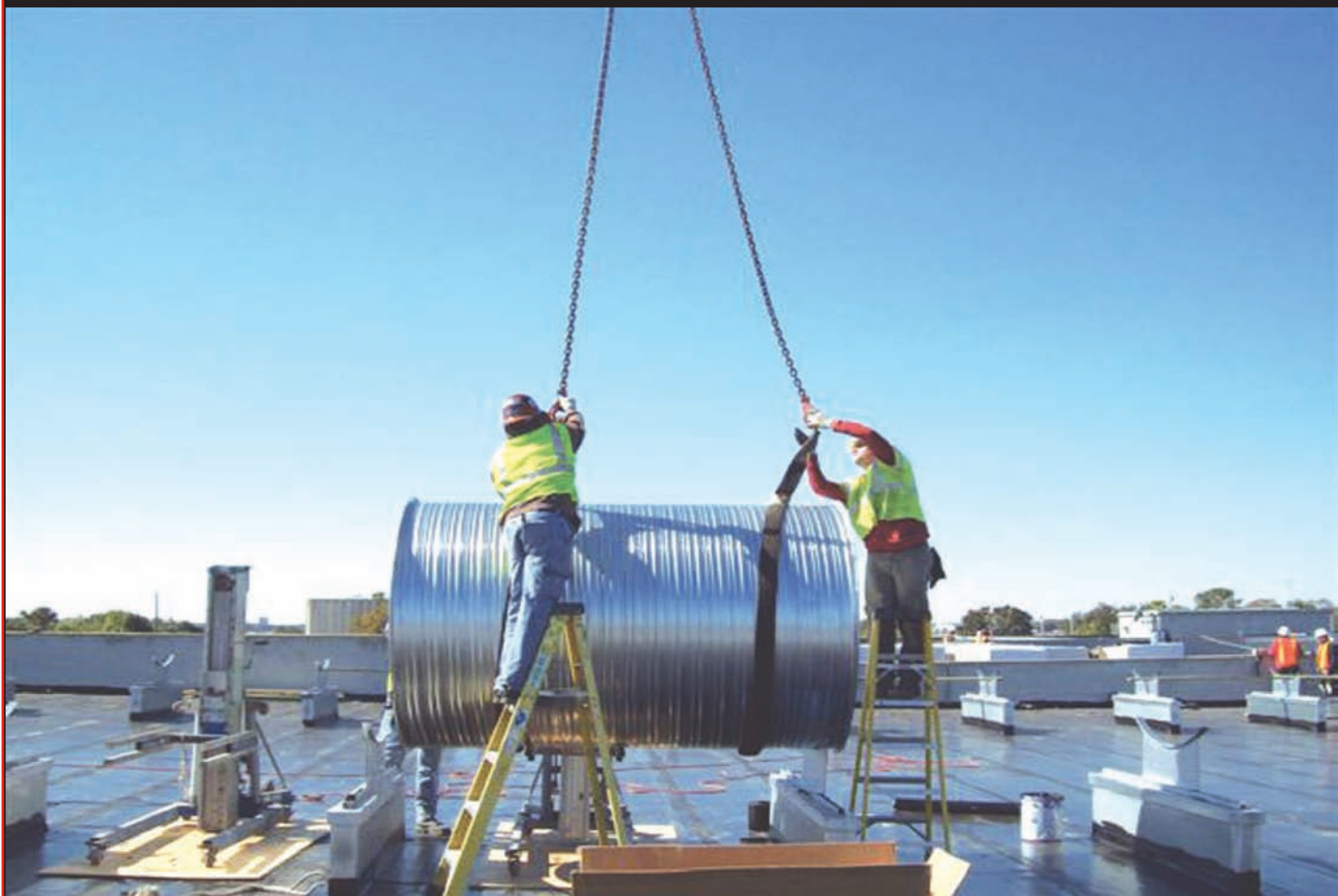
HOISTING DOUBLE WALL LINDAB SPIRAL PIPE
