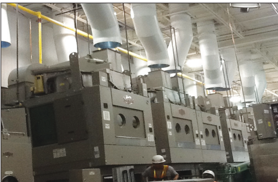
Showing duct drops with equipment set illustrating close coordination
